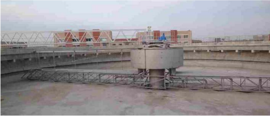
垂架式中心传动吸泥机结构示意图 Hang down posture center sucking machine structure transmission schemes
